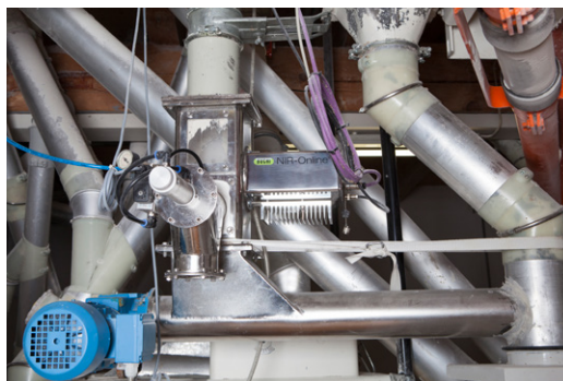
Blending optimization with NIR-Online Process Analyzer and bypass sampler.
